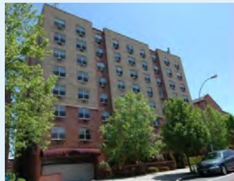
287 PROSPECT AVENUE 287 Prospect Ave., Brooklyn 53 units
